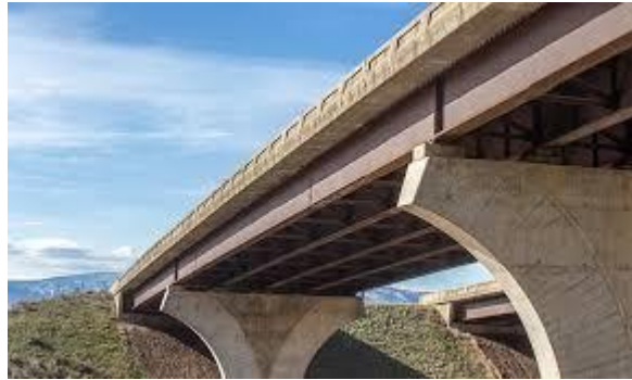
Steel Girder Bridges Beams & Plate
