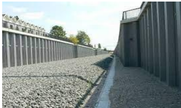
Retaining Walls Steel Piling
