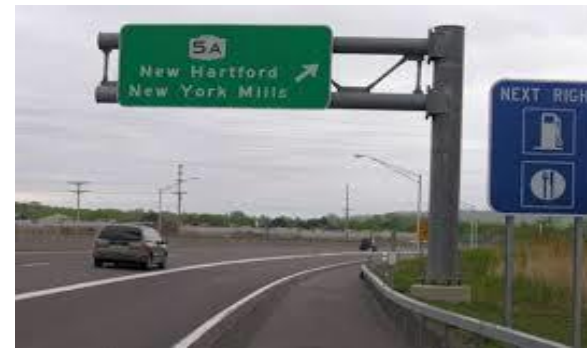
Highway Structures Steel Poles
