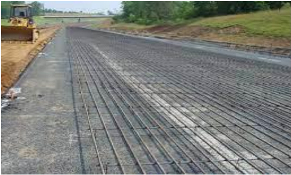
Roads Rebar & Wire Mesh
